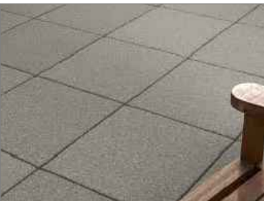
Textured concrete paving slabs to terrace
