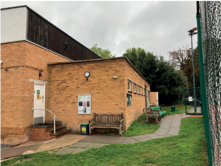
Existing changing rooms within the squash building
