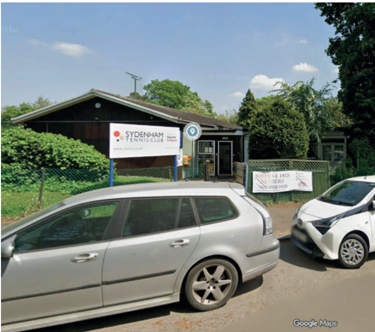
Existing clubhouse and bar
