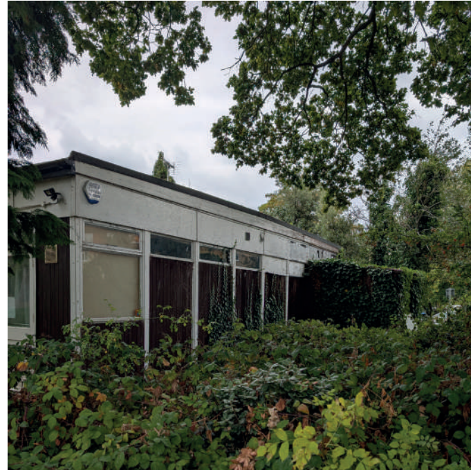
Existing Clubhouse external view - rear elevation
